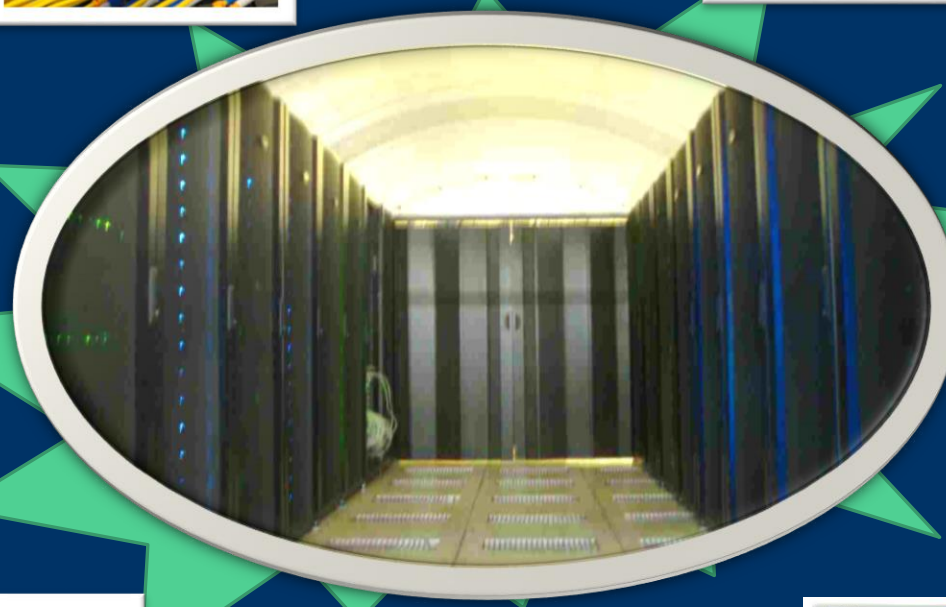
High Density Heat Containment System
